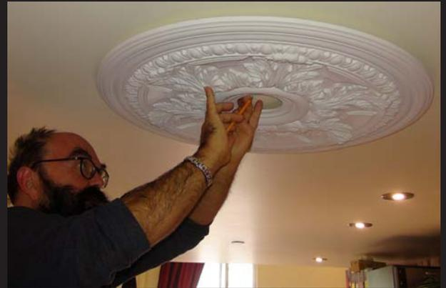
9) **Check to make sure the medallion is level on all sides. If it is not use a small wedge to pry one side downward until all sides are even. This is the time to correct any unevenness. Make sure you have pulled the wires through the center hole.**
