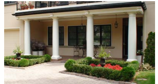
Black gutter as shown above - to be covered
