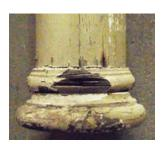
Rather than replacing the entire column we can fabricate part of the shaft plus a new load bearing Attic Base from Hardwood (White Oak, Pine, Cedar)
